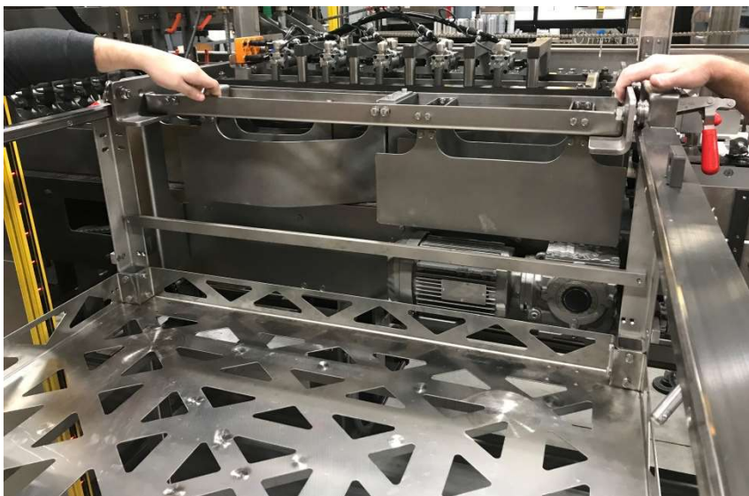
C120 - #5K - Cart In Place For Infeed Lane Cartridge Removal
